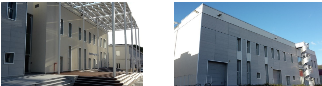
Figure 2. The Smart Energy Building (SEB).
